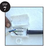
Fix the wall cover plate and secure it with the help of screws. Make sure the holes on the upper and lower part are aligned.
